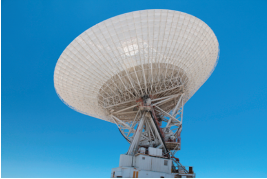
Figure 4 The Goldstone 70 m receiver dish receives weak signals from interplanetary probes far out in space that are exploring the solar system.
