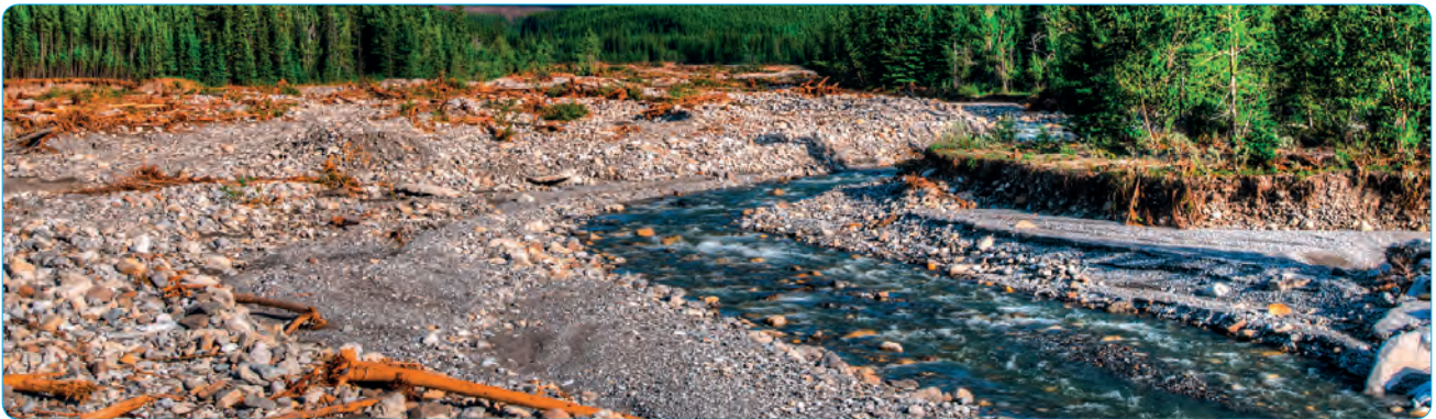
▲ Transportation: Flood waters are so powerful they can carry rocks, boulders and whole trees downstream.
