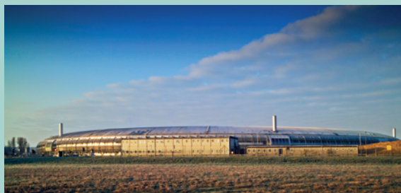
Figure A2 The Diamond Light Source (the UK's national synchrotron science facility, at Harwell in Oxfordshire) creates a very intense beam of X-rays, which scientists can use to study anything from viruses to jet engines.
