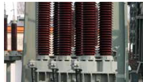
Transformers at a power station.
