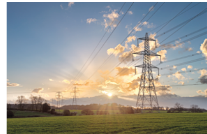
Figure 2.38: Power cables connected in the National Grid
