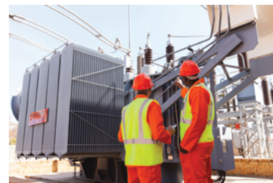
Figure 2.40: Step-up transformers are installed close to the power stations.
