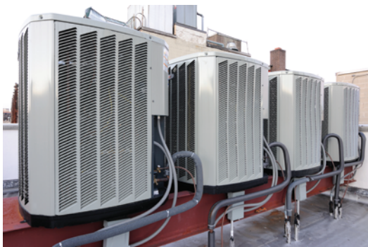
Figure 12 Air conditioners are an essential part of life in some hot areas of the world.
