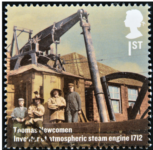
Figure 19 A postage stamp commemorating the Newcomen steam engine. In the engine, water was heated, producing steam. As the steam condensed, it pulled down a piston attached to a large wooden beam, which rocked upon a central fulcrum. The chain attachment was linked directly to a pump at the bottom of the mine.
